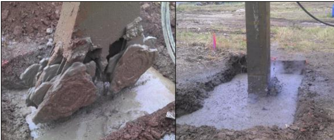
Figure 9: Execution of a CSM panel.
