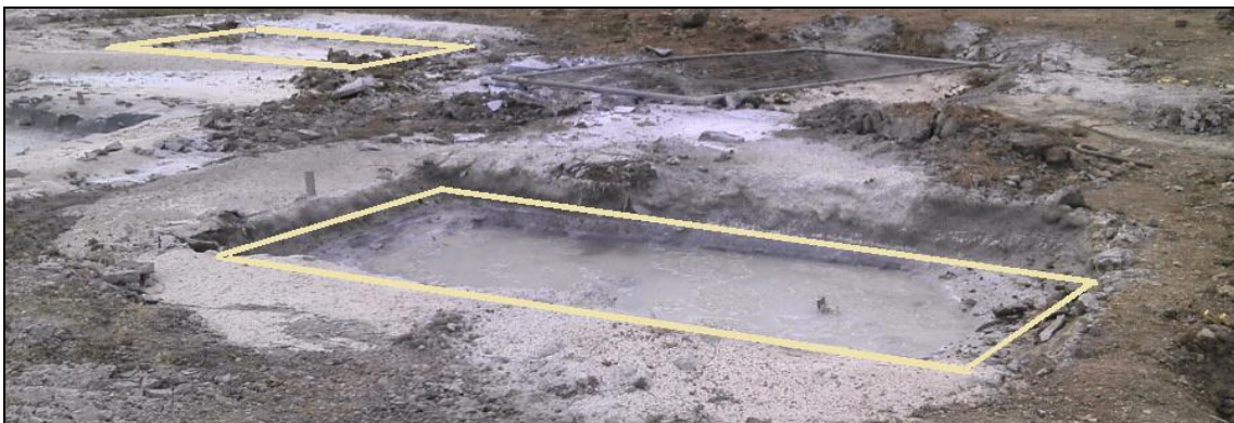
Figure 5: View of some panel caps..
