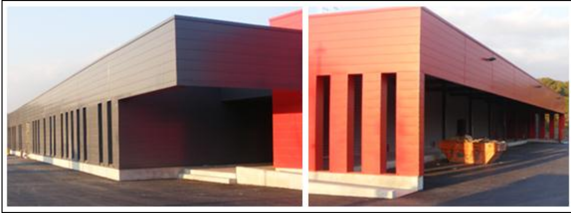
Figure 13: Views of the building after construction.
