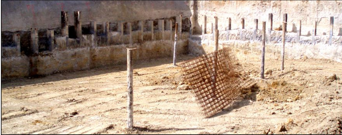
Figure 9: Foundation micropiles to the temporary support of the slab bands.
