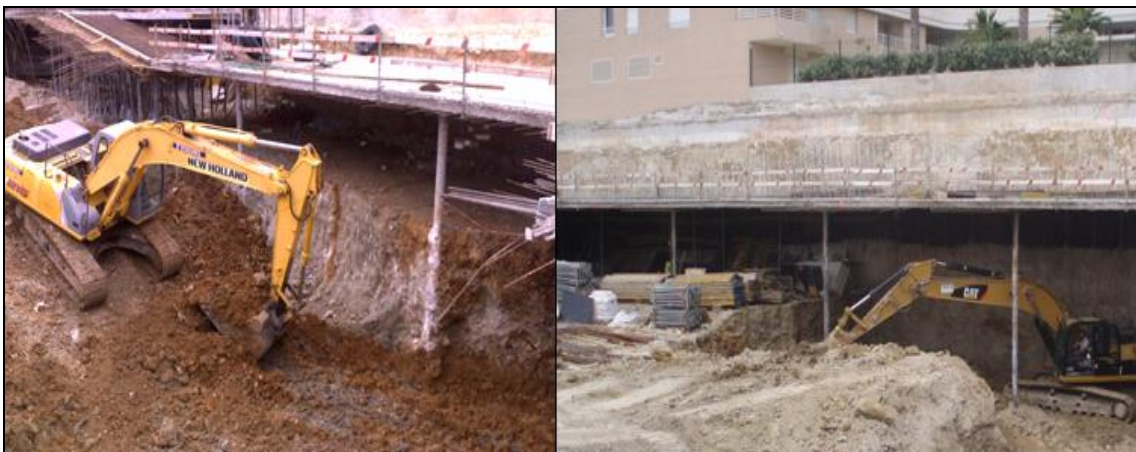
Figure 10: Views of the work during the execution of the second level of excavation.
